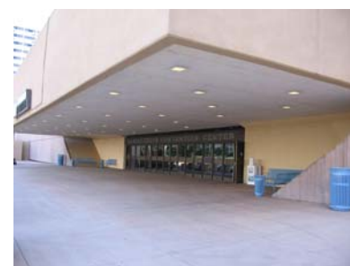
Main entrance of the Albuquerque Convention Center.
